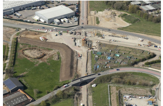
Charbridge Lane overbridge, April 2021
